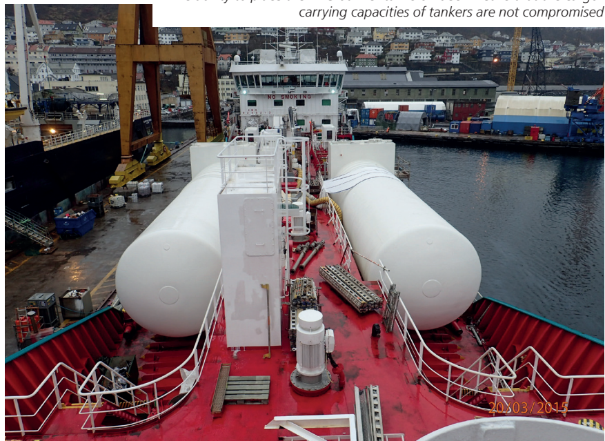
The ability to place the LNG bunker tanks on deck means that the cargo-carrying capacities of tankers are not compromised
