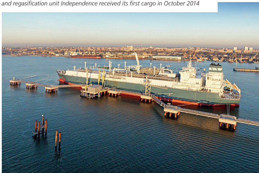
Lithuania became the world’s 30th LNG import nation when the floating storage and regasification unit Independence received its first cargo in October 2014
